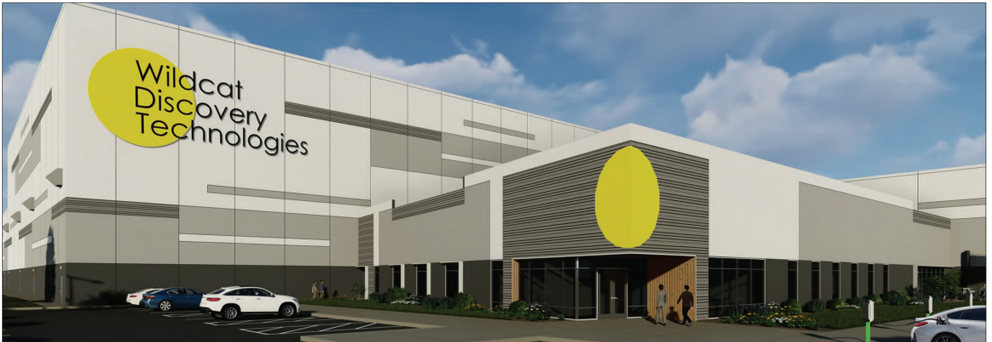
This rendering shows a 350,000-square-foot plant Wildcat Discovery Technologies plans to open in the Southeast. Rendering courtesy of Wildcat Discovery Technologies
